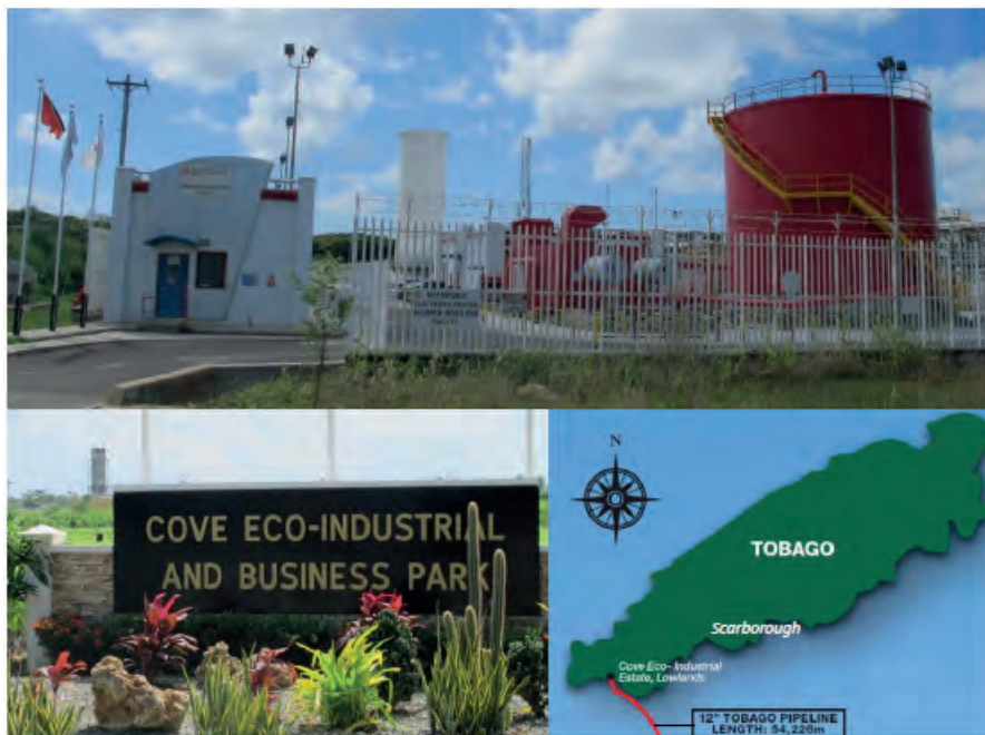
Figure 30: Tobago pipeline gas receiving plant in Cove eco-industrial estate, Tobago
