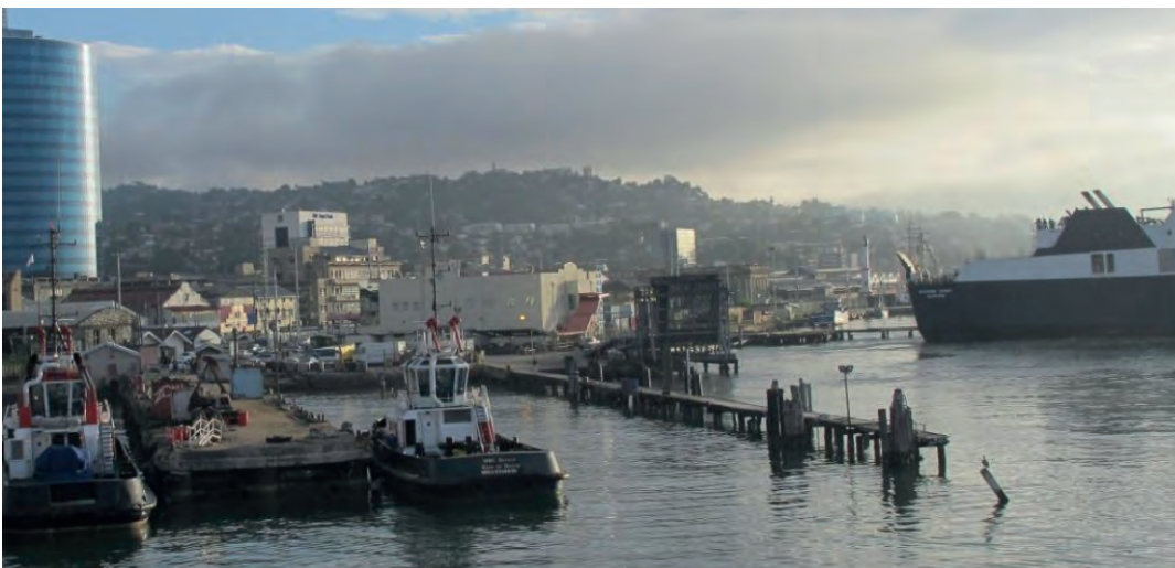
Figure 11: Port of Spain ferry terminal with St Vincent jetty (left) and terminal building (centre)
