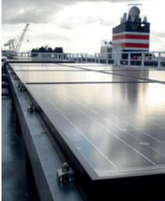
Solar panels on NYK's Auriga Leader
