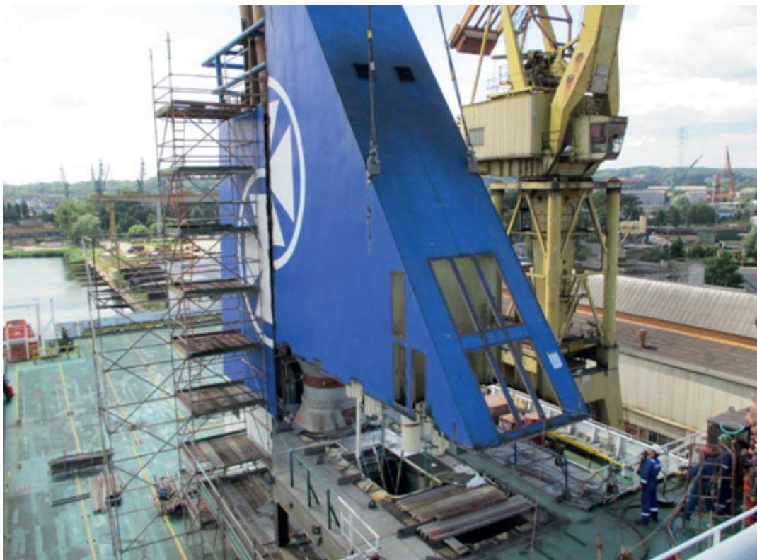
Figure 2.2: Preparations for installation of scrubber system, DFDS
